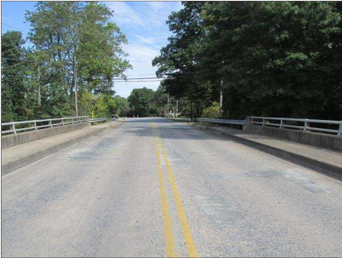
GR LOOKING WEST
