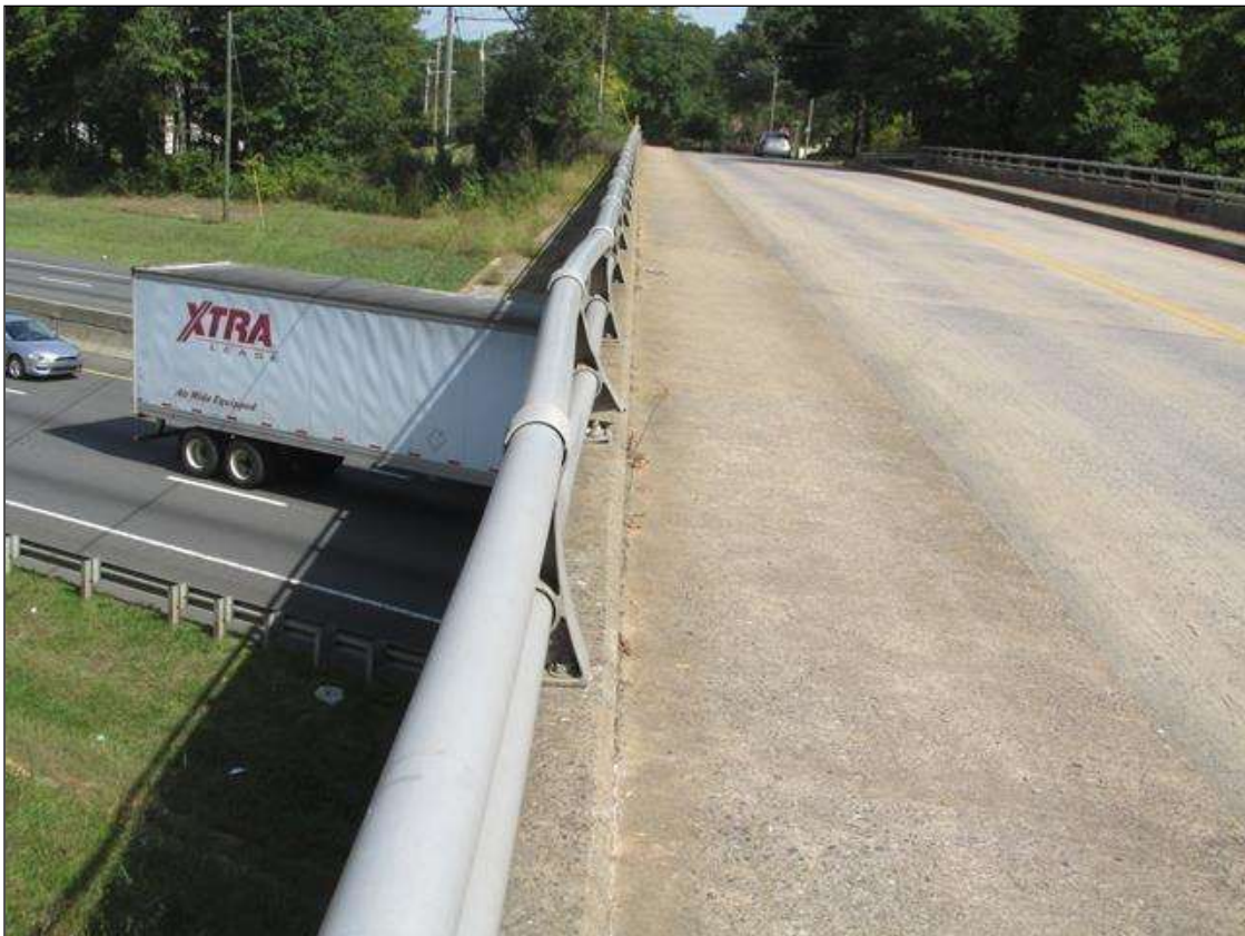
Span 4 Right Bridge Rail: 8 Feet of Distortion: Distortion not requiring mitigation of mitigated distortion.
