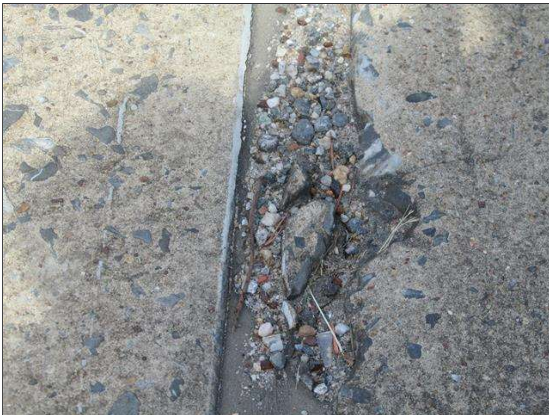
Span 1 Deck: 10 Square Feet of Cracking (RC and Other): Width greater than 0.05 in. or spacing of less than 1 ft. CHIPPING ALONG JOINT EDGES.
