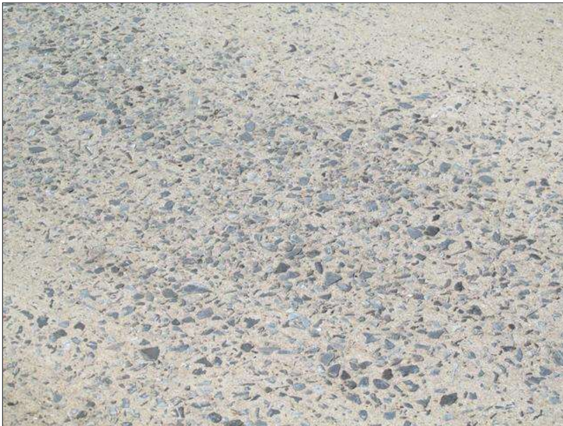
SCATTERED COARSE AGGREGATE EXPOSURE THROUGHOUT TOP OF DECK
