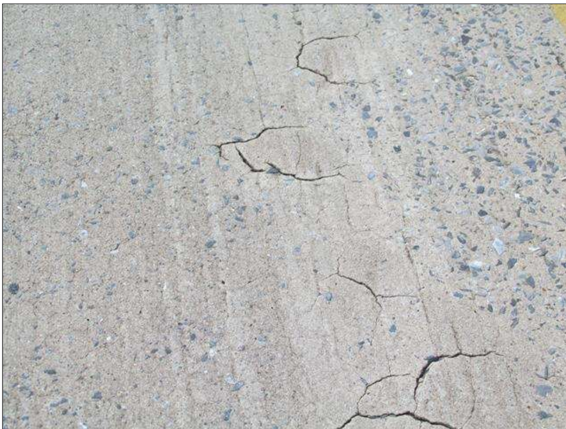
Span 2 Wearing Surface: 500 Square Feet of Crack (Wearing Surface): Width of more than 0.05 in. or spacing of less than 1.0 ft.
