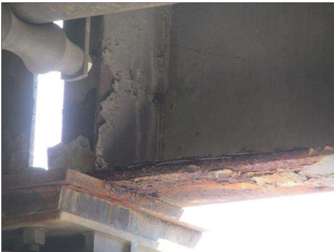
Span 1 Beam 1: 6 Feet of Corrosion: Section loss is evident or pack rust is present but does not warrant structural review.
