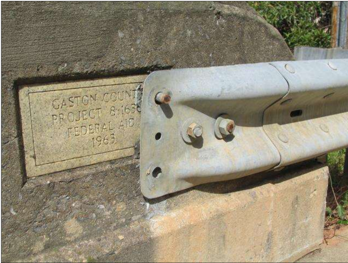
Span 1 Right Bridge Rail: 2 Feet of Connection: Missing bolts, rivets, or fasteners; broken welds; or pack rust with distortion but does not warrant a structural review. GUARDRAIL CONNECTION TO CONCRETE BRIDGE RAIL.
