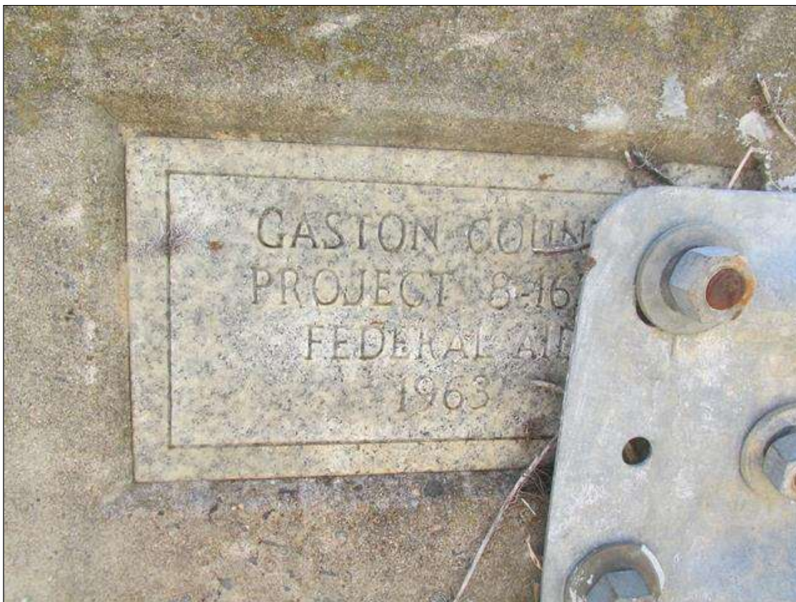
DATA PLATE, EAST APPROACH
