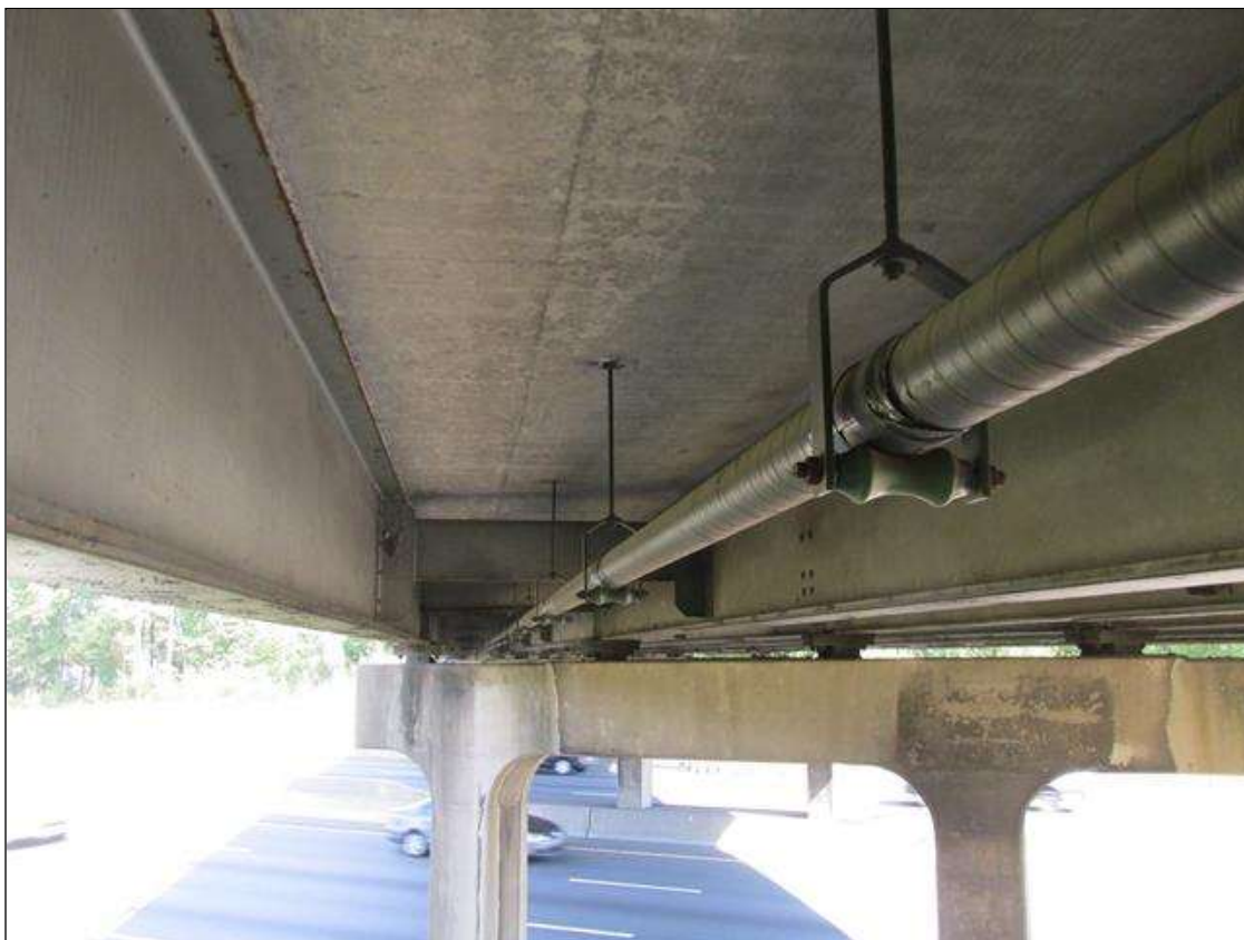
4" GAS LINE HANGING FROM STEEL SUPPORTS, BAY 5
