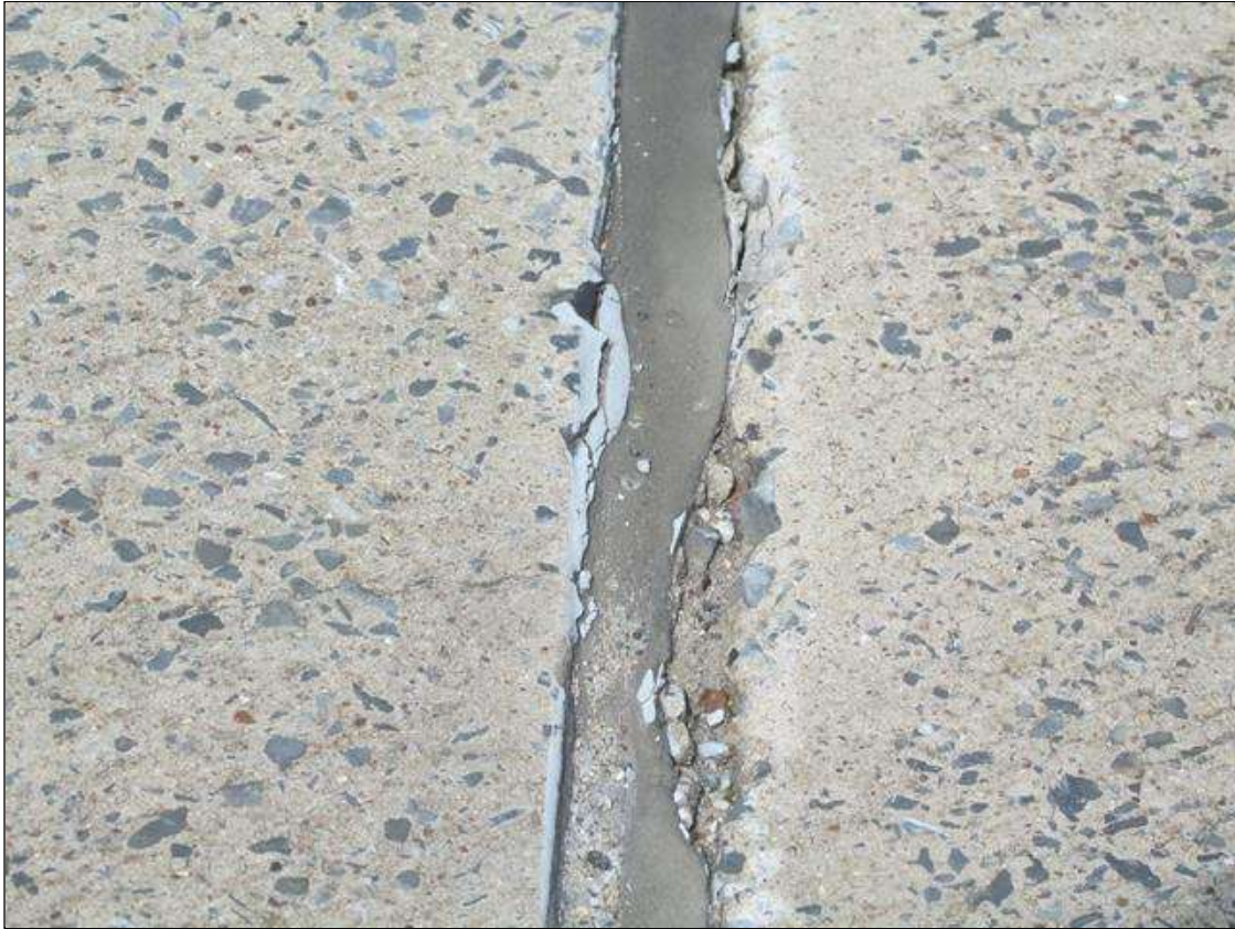
Expansion Joint 1 : 23 Feet of Seal Adhesion: Adhered for more than 50% of the joint height.
