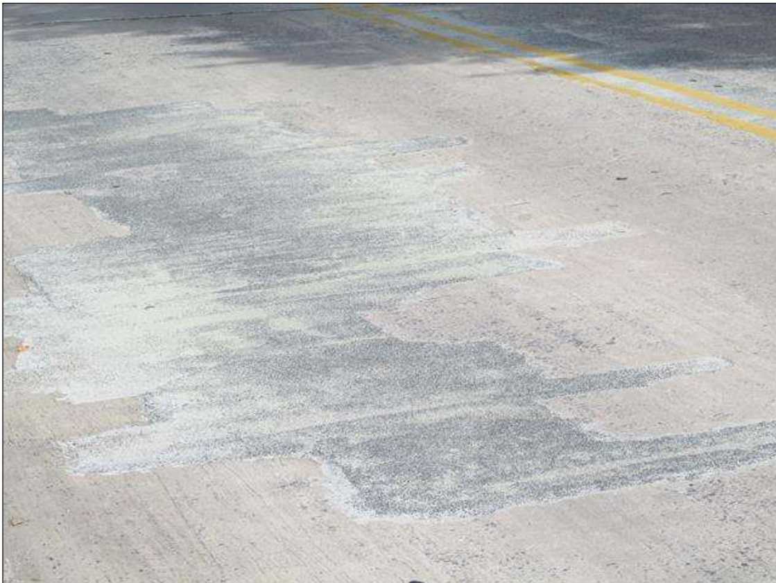
Span 1 Wearing Surface: 400 Square Feet of Delamination/Spall/Patched Area/Pothole (Wearing Surfaces): Delaminated. Spall less than 1 in. deep or less than 6 in. diameter. Patched area that is sound. Partial depth pothole.
