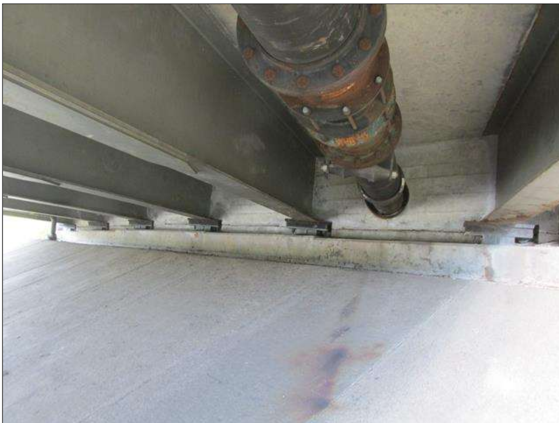
12" DIP HANGING FROM STEEL SUPPORTS, BAY 1
